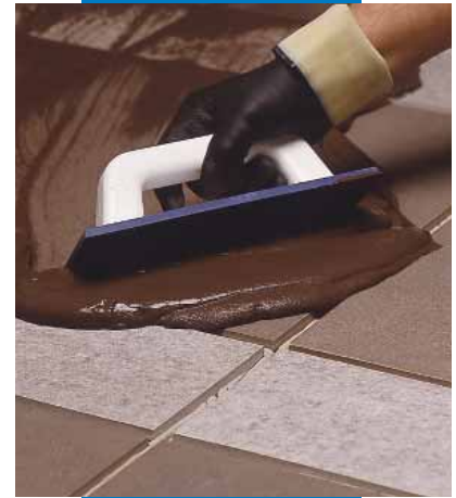
Spreading Ultracolor Plus on a floor with a rubber float
